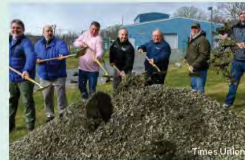
Above: Groundbreaking for new water pipeline, March 2024
