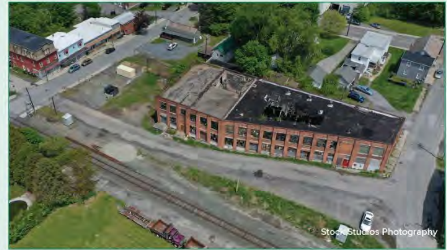
Above: Aerial image of existing site
