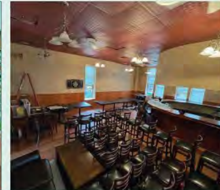
Above: Existing conditions on 2nd floor
