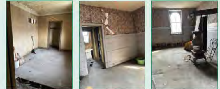
Above: Pictures of existing conditions at 3rd floor
